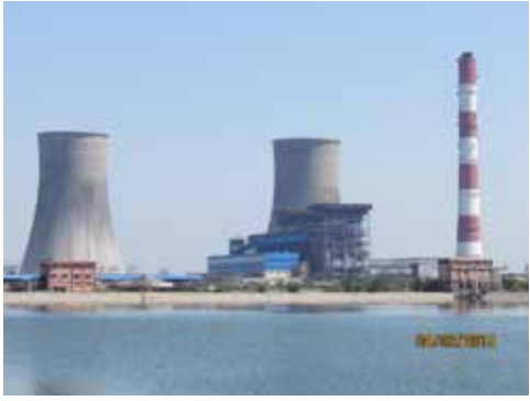
RRVUNL 2x600 MW TPP Kalisindh, Rajasthan. Unit # 2 Synchronized
